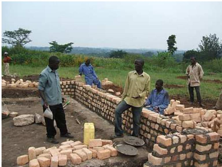
Laying bricks from foundations to slab level
