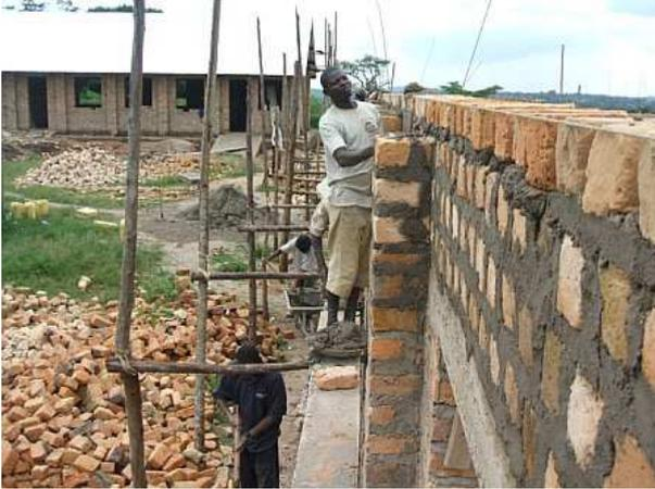
Checking line and level of brickwork at wall plate level
