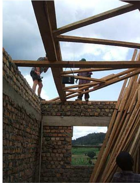
Making trusses on top of the building to avoid heavy lifting
