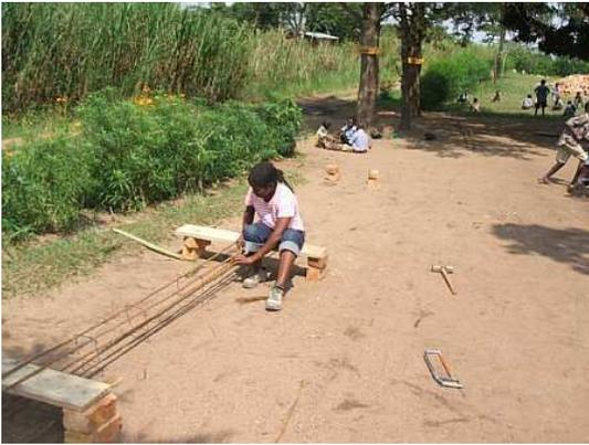
Fabricating reinforcement cage for ring beam
