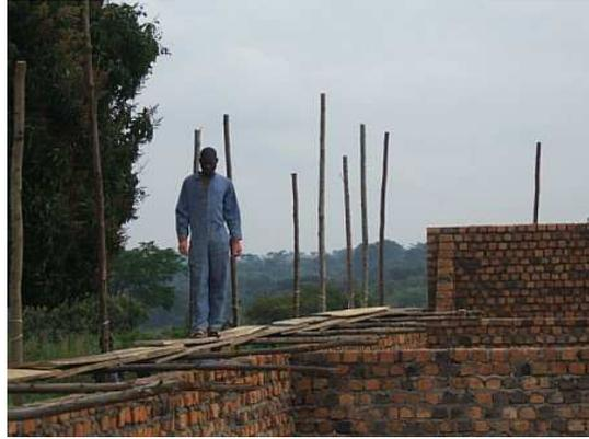
Scaffolding for bricklaying up to ring beam level
