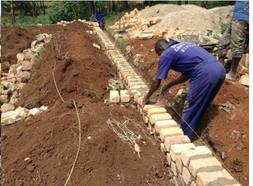
Building work in progress
