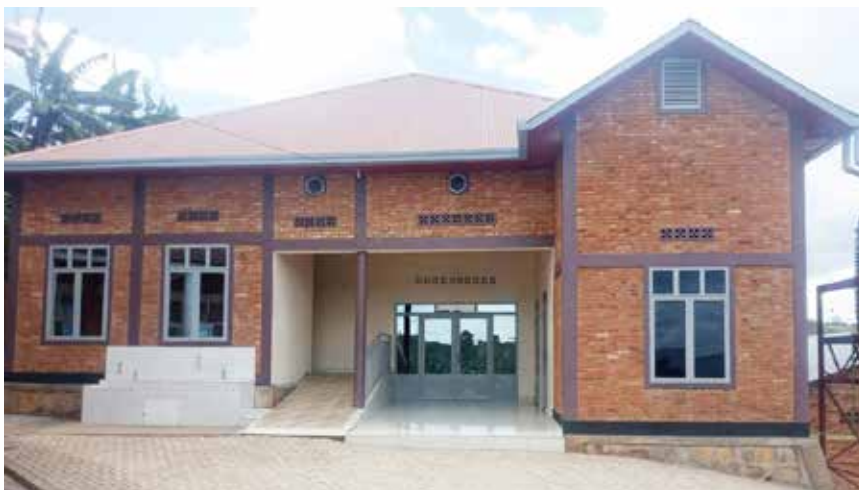
Twongerekawa Coko Co-op's new building, which houses offices, meeting rooms and bathrooms
